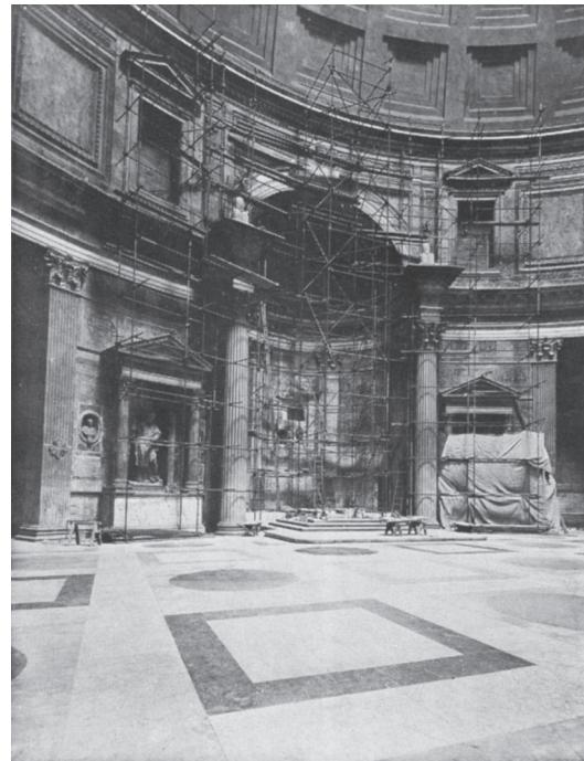
Fig. 12: Restoration of the altar niche during the 1930s (showing a section of the yet unchanged part of the attic on the right).
