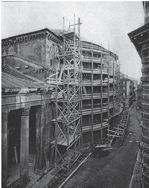
Fig. 11: Restoration work on the exterior during the 1930s.
