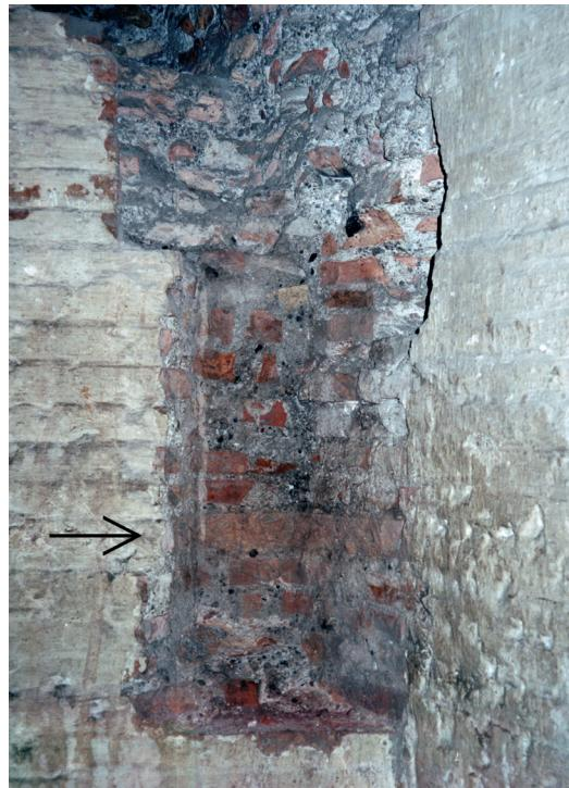
Fig. 11: Sounding no. 2 in the West Stair, second level, at the junction between the rotunda and the transitional block (author).
