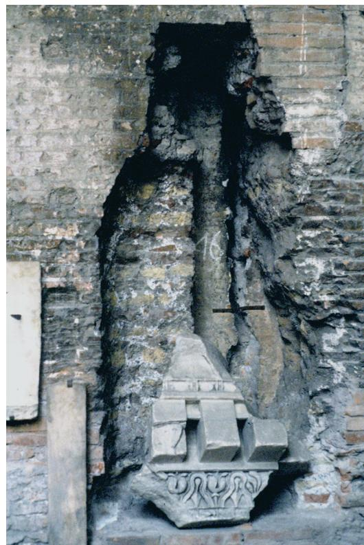
Fig. 6: The crack near the north-south axis of the Pantheon, behind the main exedra as seen from inside the *grottoni* (author).
